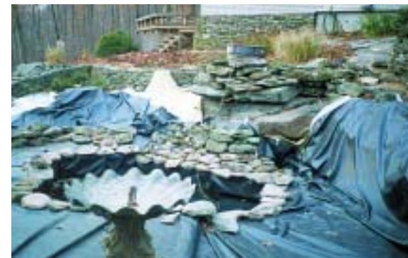
The pond excavation is fully lined.
