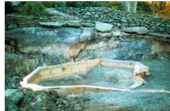
Excavating the hole for the fountain's pond required blasting.
