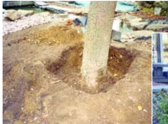
Excavate a well back down to the original soil level around the tree. The well should be wide enough to keep the mature tree trunk free of soil contact.
