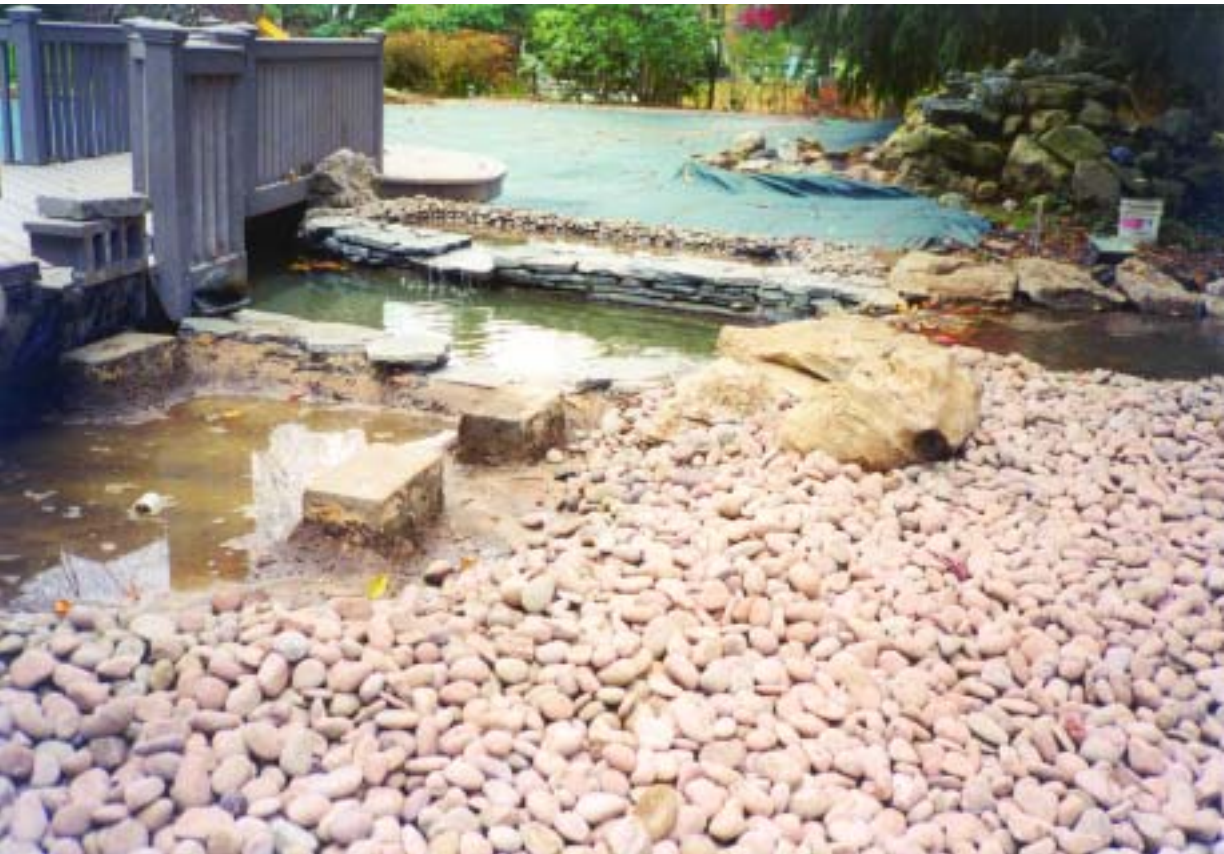
A concrete pad and a double layer of liner pieces protect the rubber liner from the weight of the concrete block supports set into the bog for the bridge.
