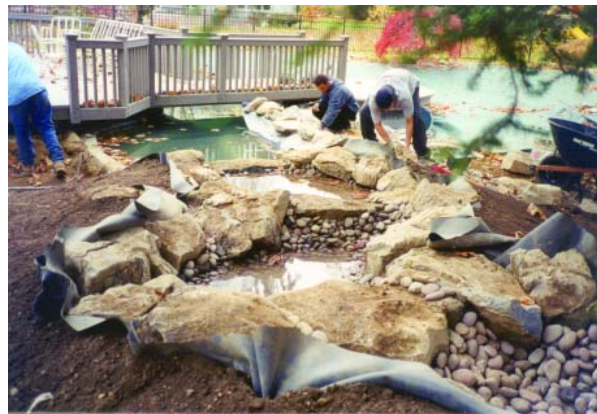
Looking toward the cabana and deck, the stream meanders from the woods. The liner will not be tucked away until we are satisfied with the stream design and its water retention.
