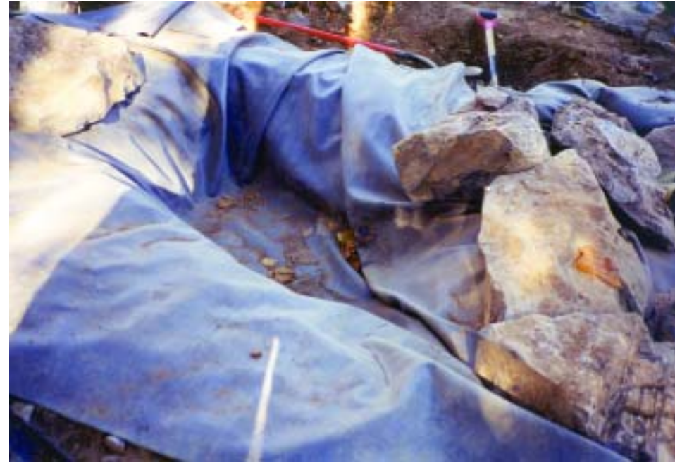
At the top of the stream, water will be cycled from the pond and filter system into a header pond that is fully lined with rubber liner.
