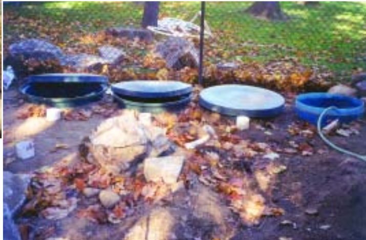
Suburban's vortex filtration system uses cone-shaped vats to effect both mechanical and biological filtration. Water enters the mechanical chamber where particulates are swirled by centrifugal action to the bottom for drainage and then flows through two chambers of bio-filter media.
