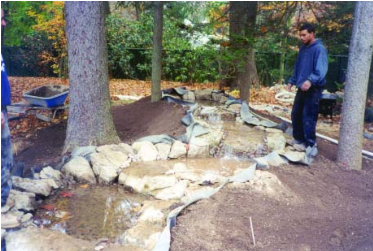
Before the stream is finished, water is run through its system to check the flow for leaks and evenness.
