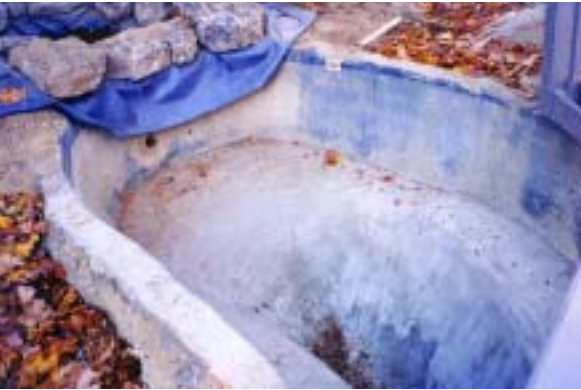
In the pond renovation, a winter drain is constructed in a shallower, separate part of the new pond near the waterfall entry from the new stream. This will allow water exchanges, if necessary, during the winter when the hibernating fish on the pond's bottom shouldn't be disturbed.
