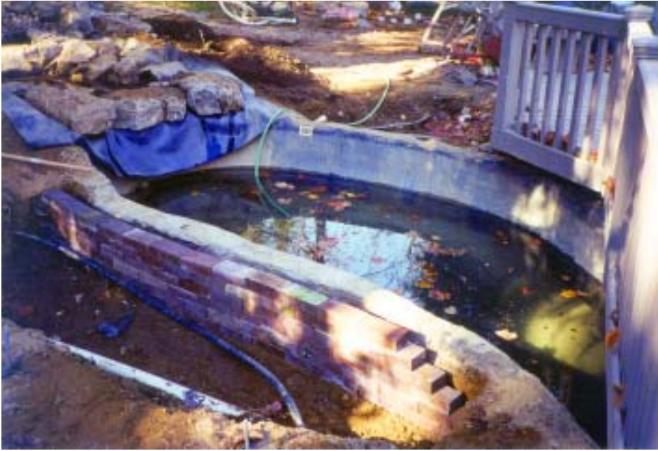
Continuing the concrete pond construction into an adjacent bog, the concrete sides are faced with bricks. This bog area is higher than the main pond's edge to allow an additional, aerating waterfall return.
