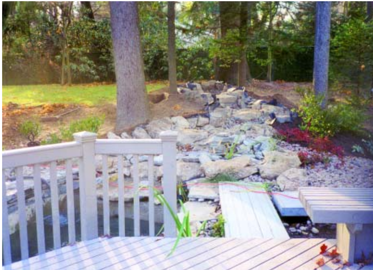
With the bridge installed, it seems a continuation of the existing deck.
