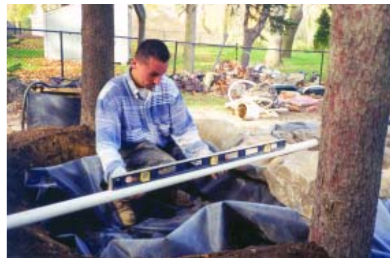
Luis, one of Suburban Water Garden's crew, checks the level side-to-side across the 4-foot-wide stream excavation. This ensures the water will run evenly through the stream bed.
