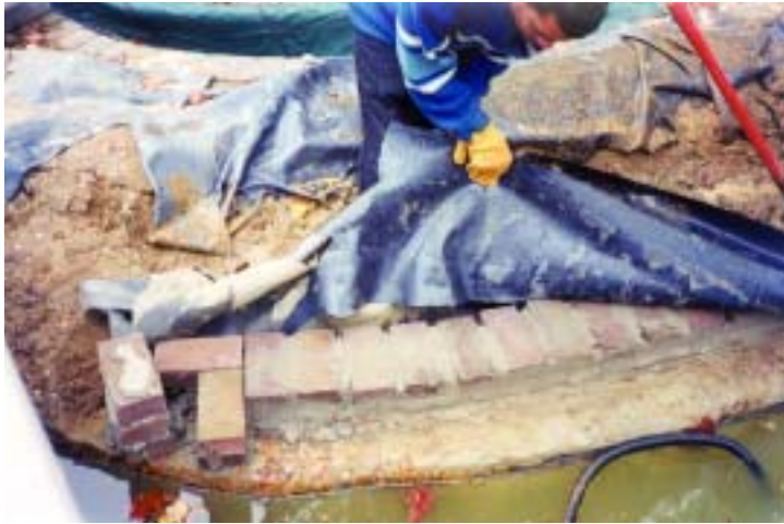
For stability, bricks are cemented into place around the edge of the shallow pond reservoir that contains the winter drain.
