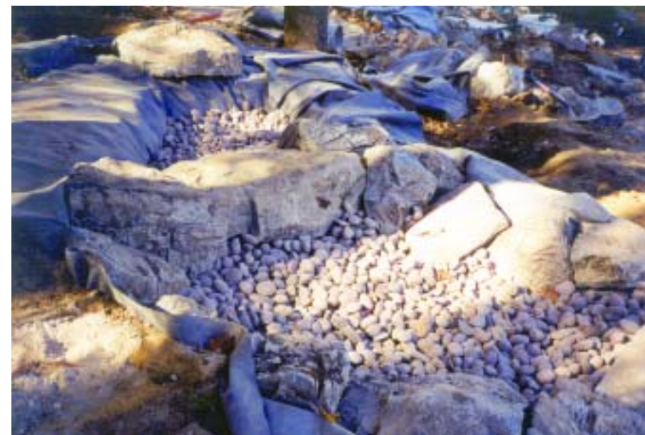
Working down the length of the stream, the soil base, sand covering, and Pocono stone is set into the bed.
