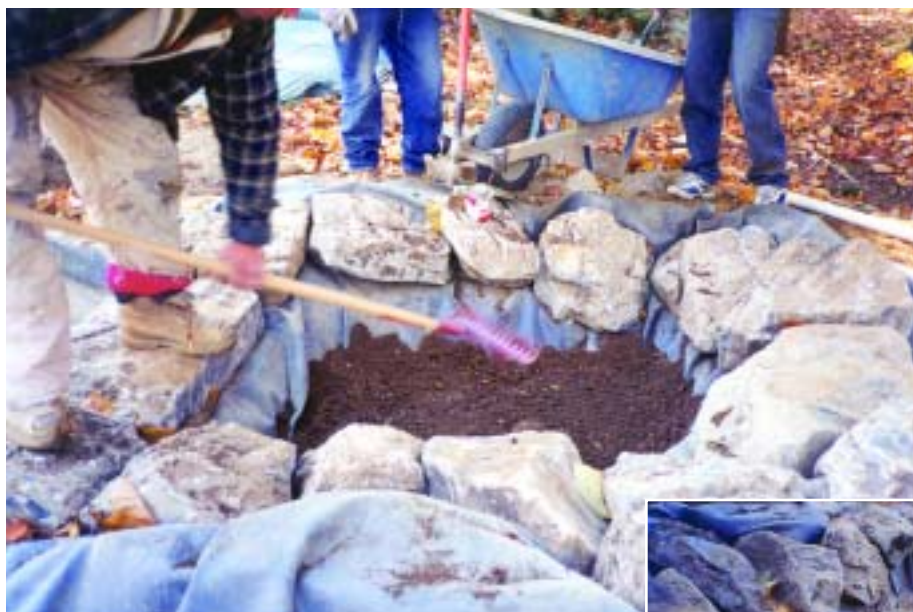
Luis smoothes the soil base in the streambed and makes certain no rocks might be present. He uses the back side of the rake to prevent puncturing the liner.
