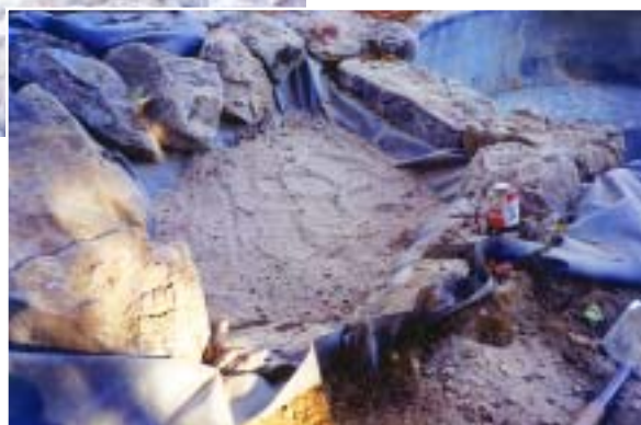
A layer of damp sand covers the soil base in the streambed. improve the circulation to the pond and eliminate any dead areas where harmful bacteria can grow.
