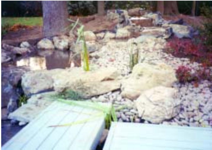
A finishing detail after the bridge is installed: Pocono stone as an aesthetic and low-maintenance ground cover accented by a trio of boulders.
